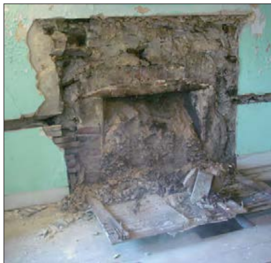
Figure 11 Image of the interior of the fireplace once the plaster and lath was removed.
