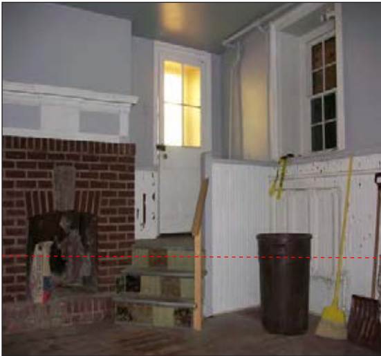
Figure 1 Red line indicates original floor height, 2010.
