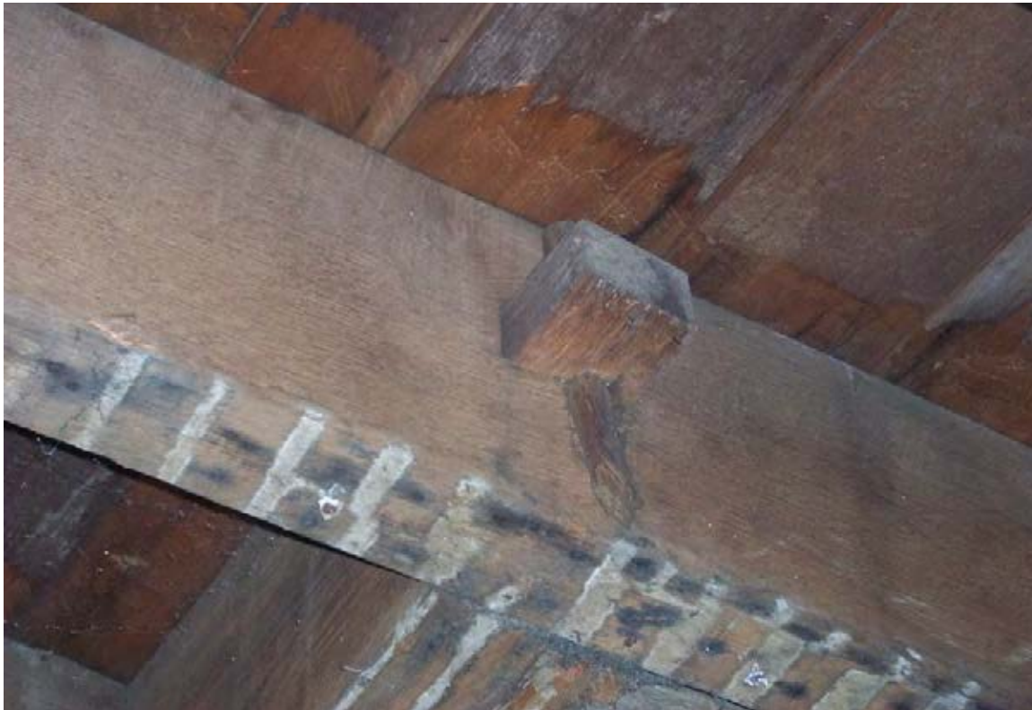
This mortise and tenon joint with peg is used to in-fill the staircase opening.
