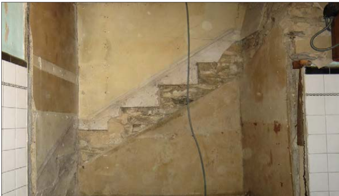
Figure 10 "In this image shows the outline of a stairway in the east plaster wall of room 203 in the west addition."
