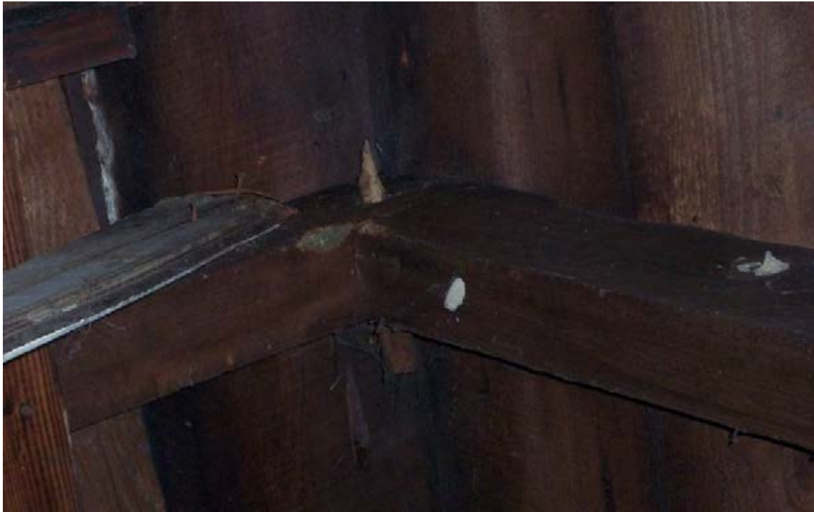
The roof rafters are connected at the ridge by a bridled joint and peg.
