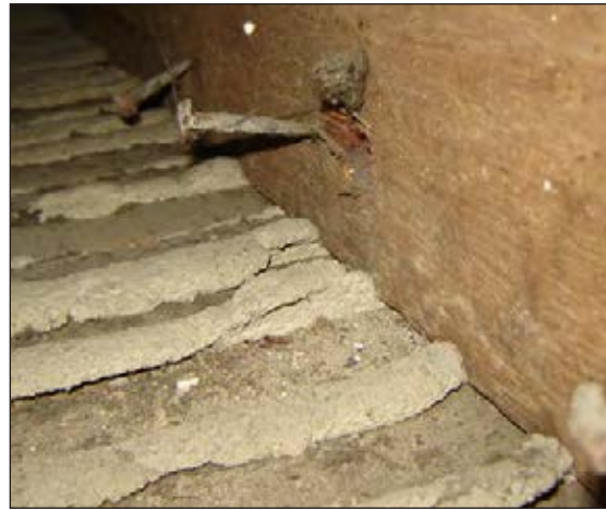
Figures 8 & 9 These images show two features of the 3rd floor joists of the west addition. Along the sides of the joists there are rows of cut nails with hand wrought heads. There are also oak pegs with a diameter of about \frac{1}{4} .
