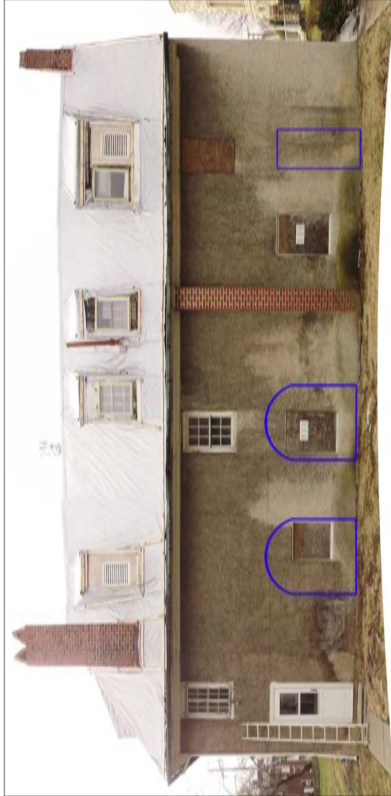
Figure 4 This image of the eastern façade, displays two brick arches and one filled in doorway. The first arch from the left could have served as a doorway leading from Sellers Hall to a breezeway, however its low apex makes this assumption problematic. The second arch from the left is also above a window and could have been included to support the weight of the wall when the window was installed. Finally, a filled in doorway was discovered on the northern end of the eastern façade. This entrance could have allowed for passage from Sellers Hall into an outbuilding that butted against Sellers Hall and the breezeway.
