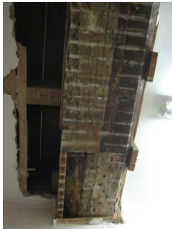
Chamfered section of the summer beam, 2010.
