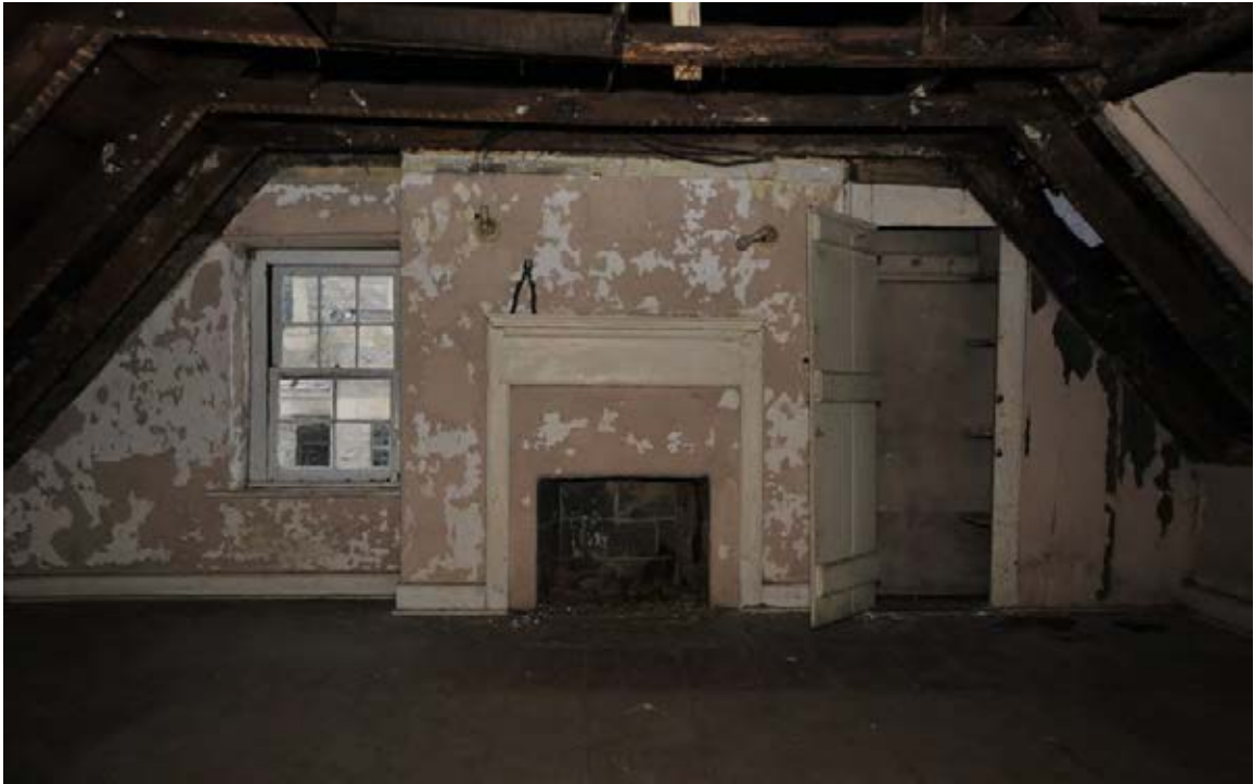
Figure 13 Room 306b, north wall, 2010.
