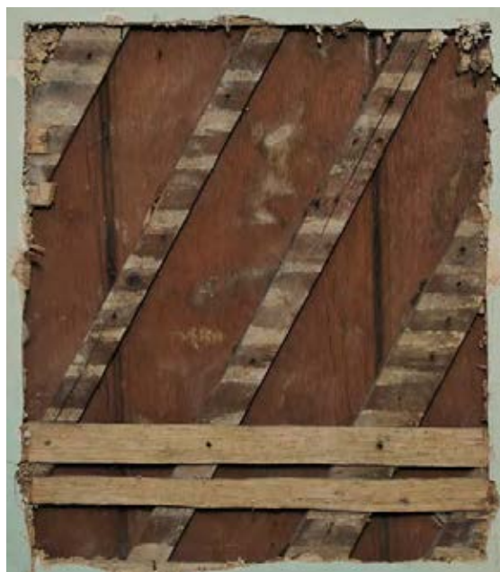
Figure 1 Wood Board Partitions from the East, 2010.
