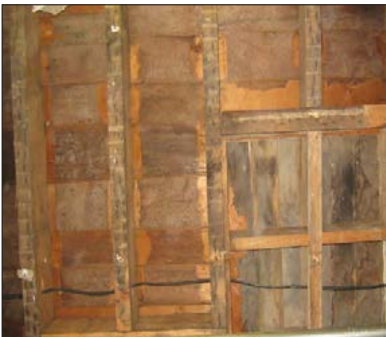
Figure 3 Framed opening in room 106, 2010.
