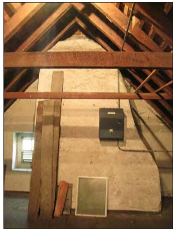
Figure 3 The chimney at Varnum's Quarters, visible on the third floor.
