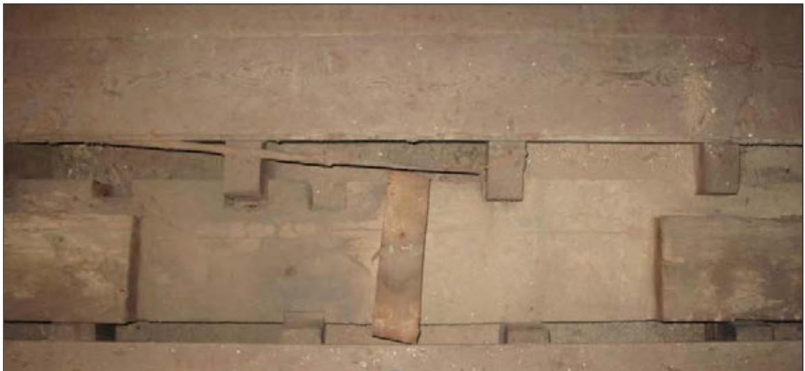
Figure 8 The notch cut into the summer beam indicates the original placement of the hearth in the room.
