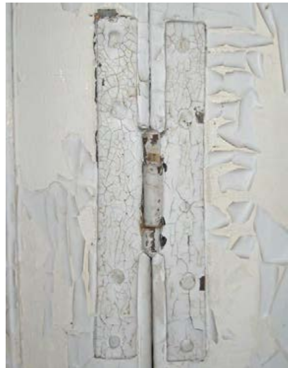
Figure 8 Photograph of H-hinge, popular during the 18th century.
