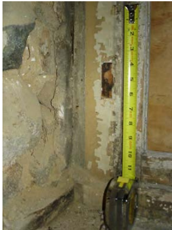
Figure 3 Photograph of window NID detail.
