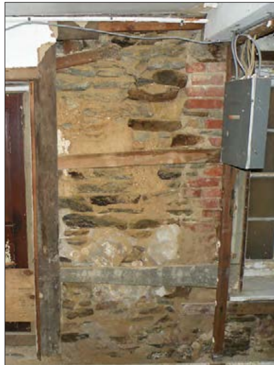
Figure 2 "A vertical patch of bricks in the 1st floor west wall of the west addition shows where the north wall of building A was removed."
