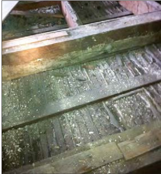
Figure 9 White wash on the underside of a beam on the third floor showing where the fireplace on the floor underneath would have been.
