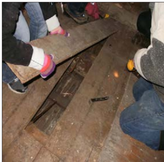
Figure 8 Removal of floor boards in room 302, 2010.
