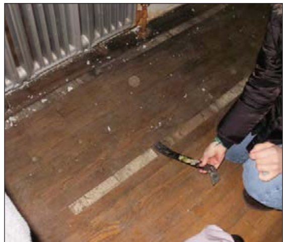
Figure 4 Removal of modern strip flooring in room 202, 2010.
