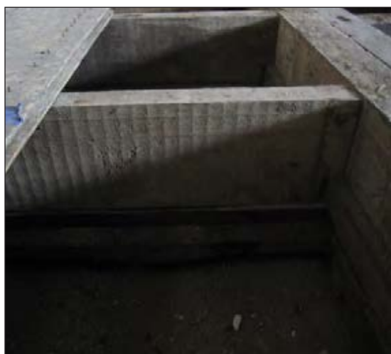
Figure 14 Vertical sawmill marks, 2010.
