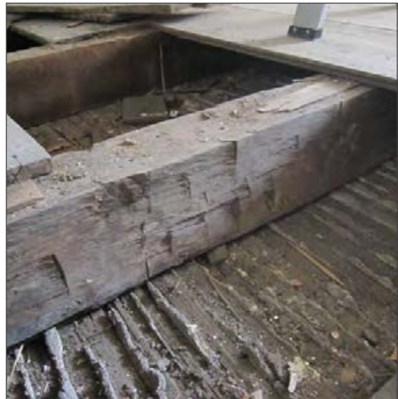
Figure 1 Hand hewn joist room 302, 2010.
