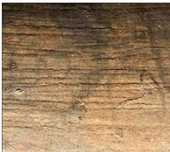
Figure 13 Pit saw marks, 2010.
