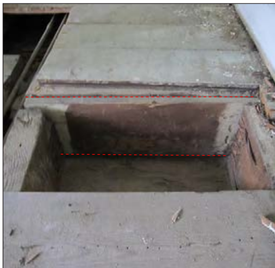
Figure 7 Original stair riser on summer beam in room 201, 2010.
