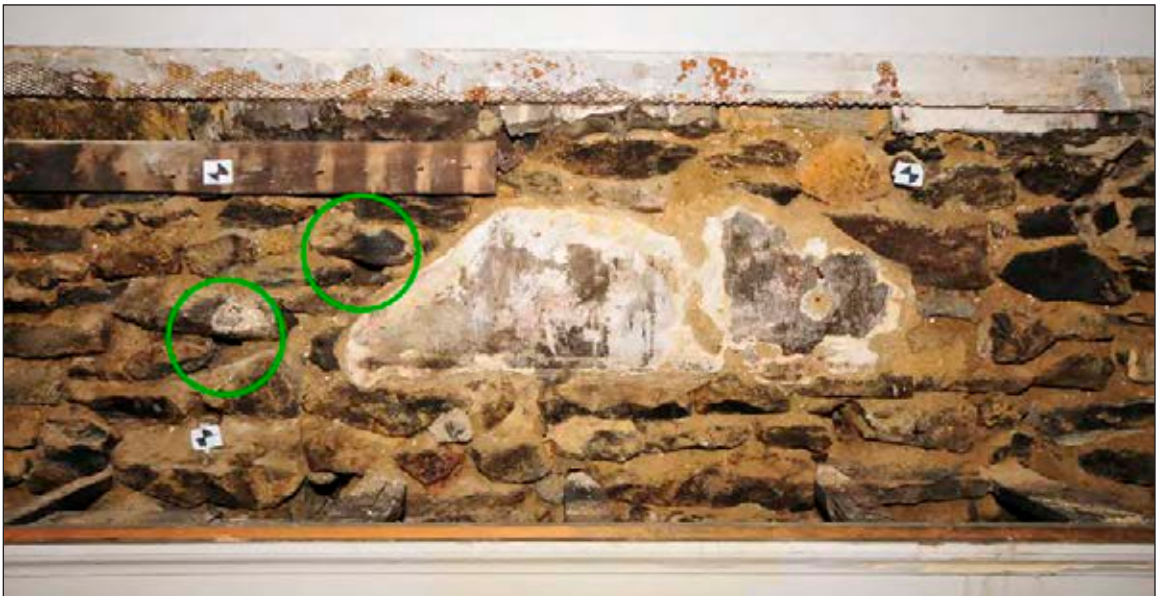
Figure 3 Interior elevation of east wall, exhibiting staircase evidence, 2010.
