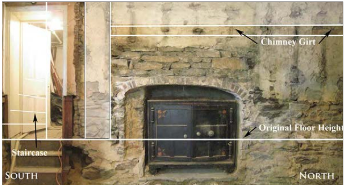
Figure 2 This image shows where the cooking fireplace would have been positioned in 1680. The extant wall would have been the back of the stairwell and the fireplace and the structures would have extended approximately 4 ft into the room.
