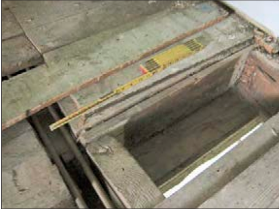
Figure 8 Riser board attached to the summer beam, view from second floor, 2010.
