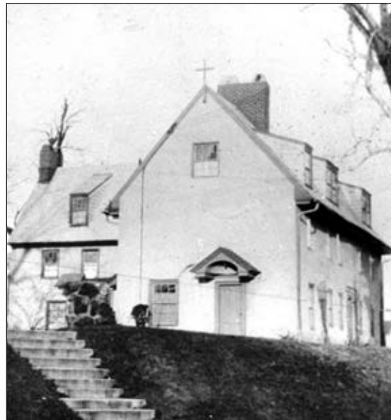
Figure 12 “West end of Sellers Hall in the 1930s showing the west addition seamlessly blended with the rest of Sellers Hall with a layer of stucco”
