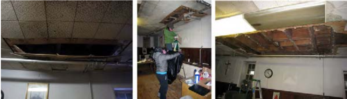
Figure 1 Framing of Rm 106; before, during and after ceiling removal, 2010.
