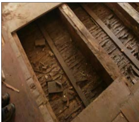
Figure 9 Floor Joists running north/south in room 302, 2010.
