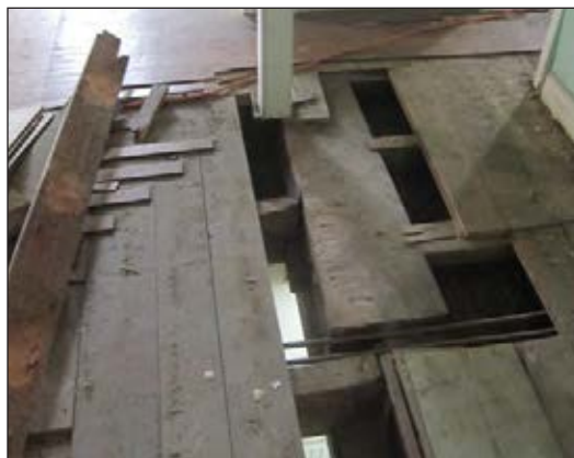
Figure 6 Summer beam in room 201, 2010.
