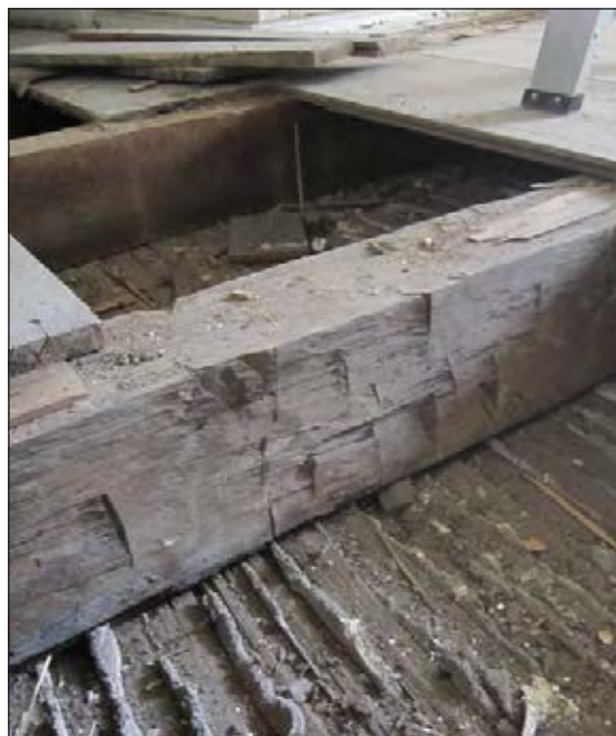
Figure 12 Hand hewn joist room 302, 2010.
