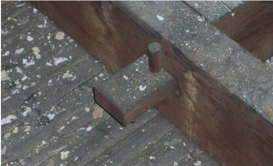
This is an example of a later mortise and tenon joint with peg. The original mortise and tenons have a diminishing shoulder, or slant, above the tenon. This method reduced the amount of material cut, providing for a stronger tenon.
