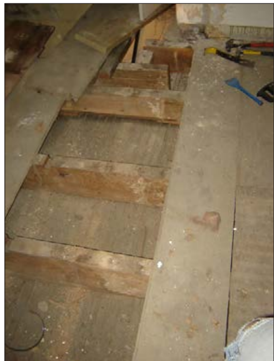
Figure 7 Third floor joists of the west addition: Faint vertical lines of paint can be seen on the joists in this picture. These lines represent where the joists passed through the former north wall of building A”
