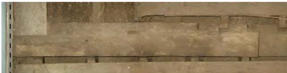
Photo rectified to top of beam only Matt Wicklund
