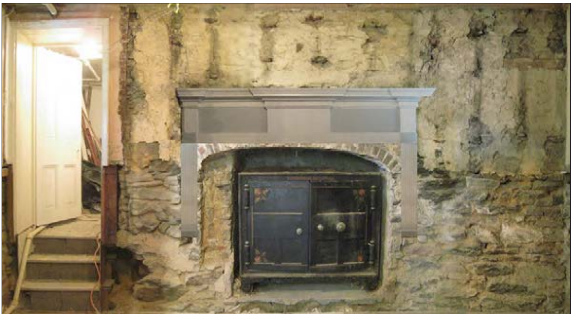
Figure 6 Image of the mantel with leg height at the original floor level using the molding profile of the first floor east fireplace which resembles the mantel in the photograph.
