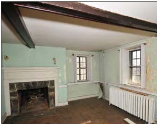
Figure 10 Room 201, southeast corner, 2010.
