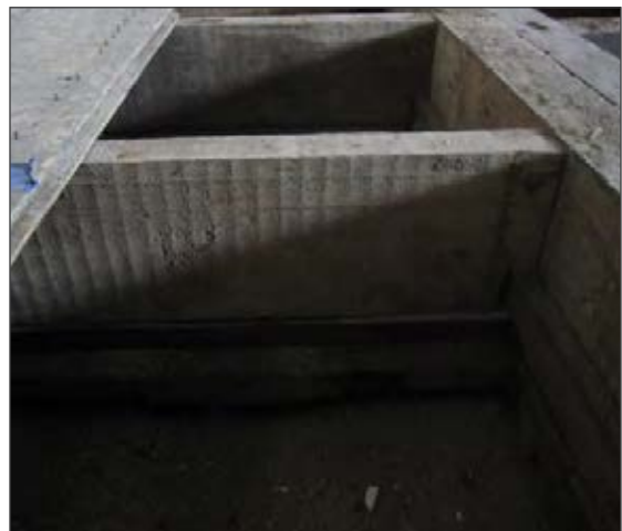
Figure 3 Vertical sawmill marks, 2010.
