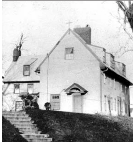
Figure 2 West end of Sellers Hall in the 1930s showing the west addition seamlessly blended with the rest of Sellers Hall with a layer of stucco.
