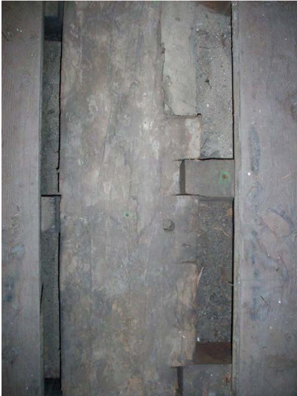
Original joists, pictured on the left of the chimney girt, are cogged with a diminishing shoulder. There are no pockets cut into the chimney girt on the opposite side, the west side, where it would've abutted the masonry of the original cooking chimney. Joists on the left side are resting on cleats.
