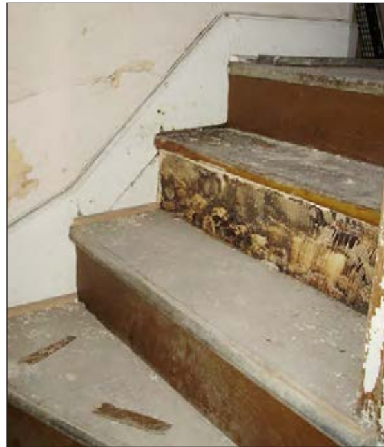
Figure 5 Three original steps at the top of the stairs on the third floor, 2010.
