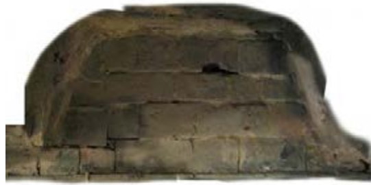
Figure 10 The firebox floor is original the fireplace location and is made of irregularly shaped handmade bricks.
