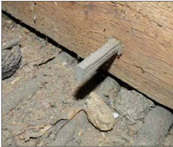
Figures 8 & 9 These images show two features of the 3rd floor joists of the west addition. Along the sides of the joists there are rows of cut nails with hand wrought heads. There are also oak pegs with a diameter of about \frac{1}{4} .
