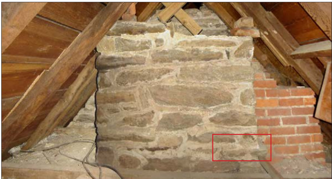
Figure 3 “The stack of the west chimney features a projecting flat stone at the lower right side of the stone work. This was a flashing course to shed water away from a former roof for building A that abutted the chimney”
