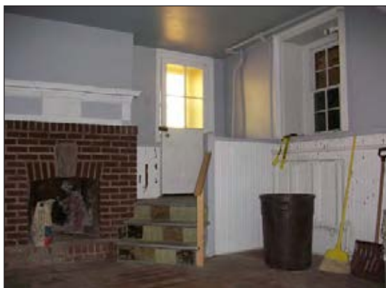
Figure 7 Room 101, southeast entry, 2010.
