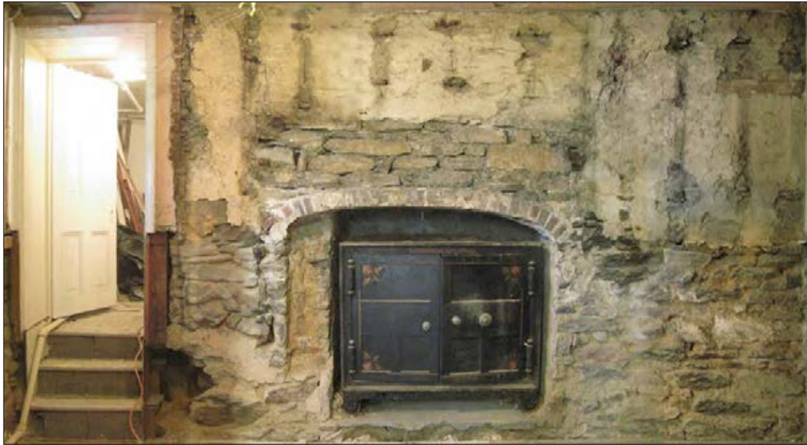
Figure 4 Elevation of west wall, in Rm 102. The brick arch of the firebox and north cove can still be seen.
