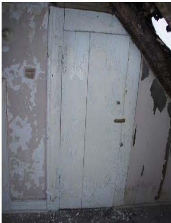
Figure 7 Photograph of late 17th-/early-18th century, plain and batten door.
