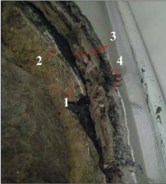
Figure 7 The stratigraphies of finishes on the fireplace in room 106: substrate: schist; layer one: brown coat, scratch coat and finish coat of plaster; layer two: scratch coat and finish coat of plaster; layer three: vegetable board, fiber board and plaster; layer four metal lath, scratch coat and finish coat of plaster.
