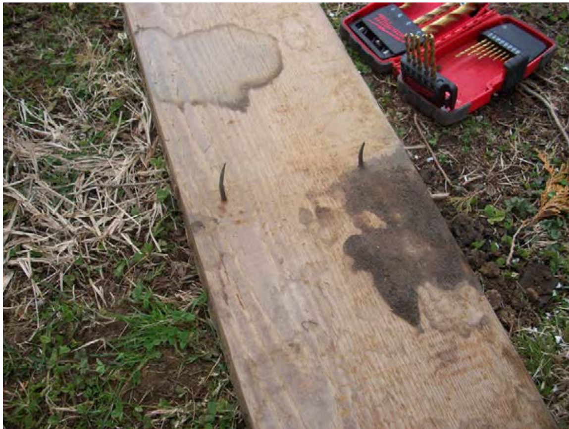
Figure 8 The interior side of the soffit board after removal. The wood is hand planed and the nails are hand wrought.
