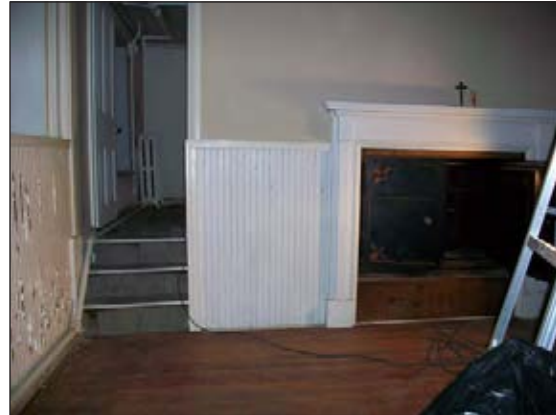
Figure 8: Room 102 showing safe-filled fireplace and stairs into Room 103, 2010.
