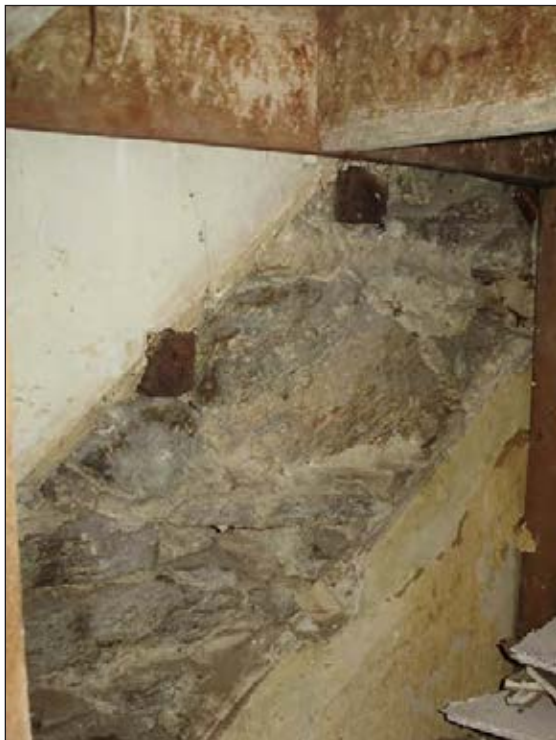
Figure 6: Plaster outline below the current stairs on the third floor, 2010.
