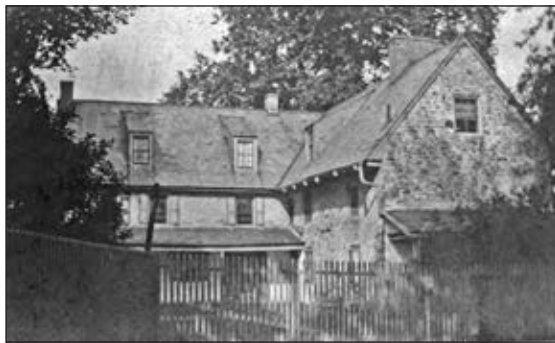
Figure 11 West end of Sellers Hall in the 1890s showing the complete west addition without stucco.
