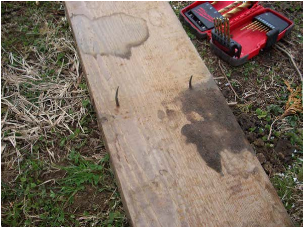
Figure 1 The soffit board of the original cornice.
