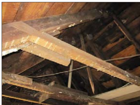
Figure 16 Roofing system - rafters and collar ties, room 301, 2010.
