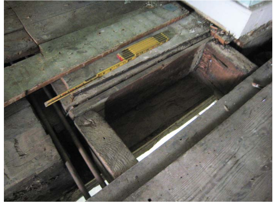
RISER BOARD ATTACHED TO THE SUMMER BEAM, VIEW FROM SECOND FLOOR, 2010.
