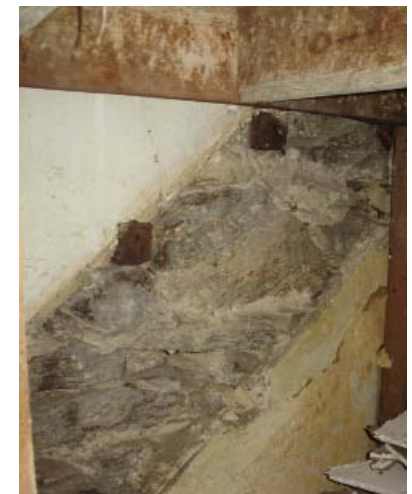
PLASTER OUTLINE BELOW THE CURRENT STAIRS, 2010.
