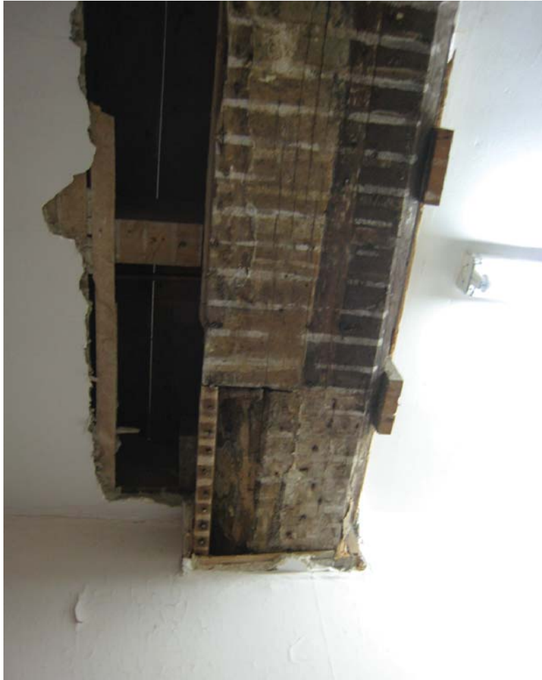
CHAMFERED SECTION OF THE SUMMER BEAM, 2010.
