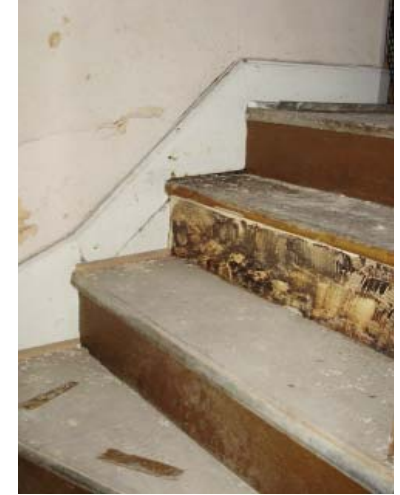
THIRD FLOOR: THREE ORIGINAL STEPS
