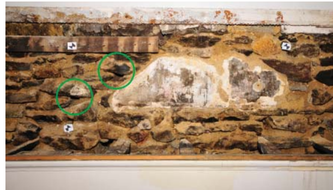
INTERIOR ELEVATION OF EAST WALL, EXHIBITING STAIRCASE EVIDENCE, 2010.
