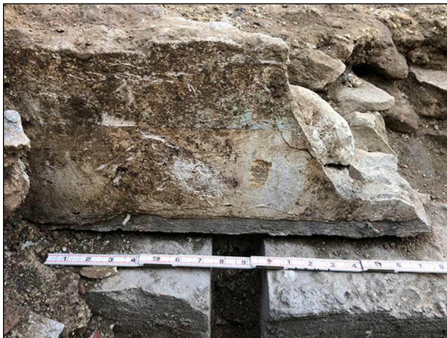
Photograph 6. Concrete pier and plaster detail, view east.
