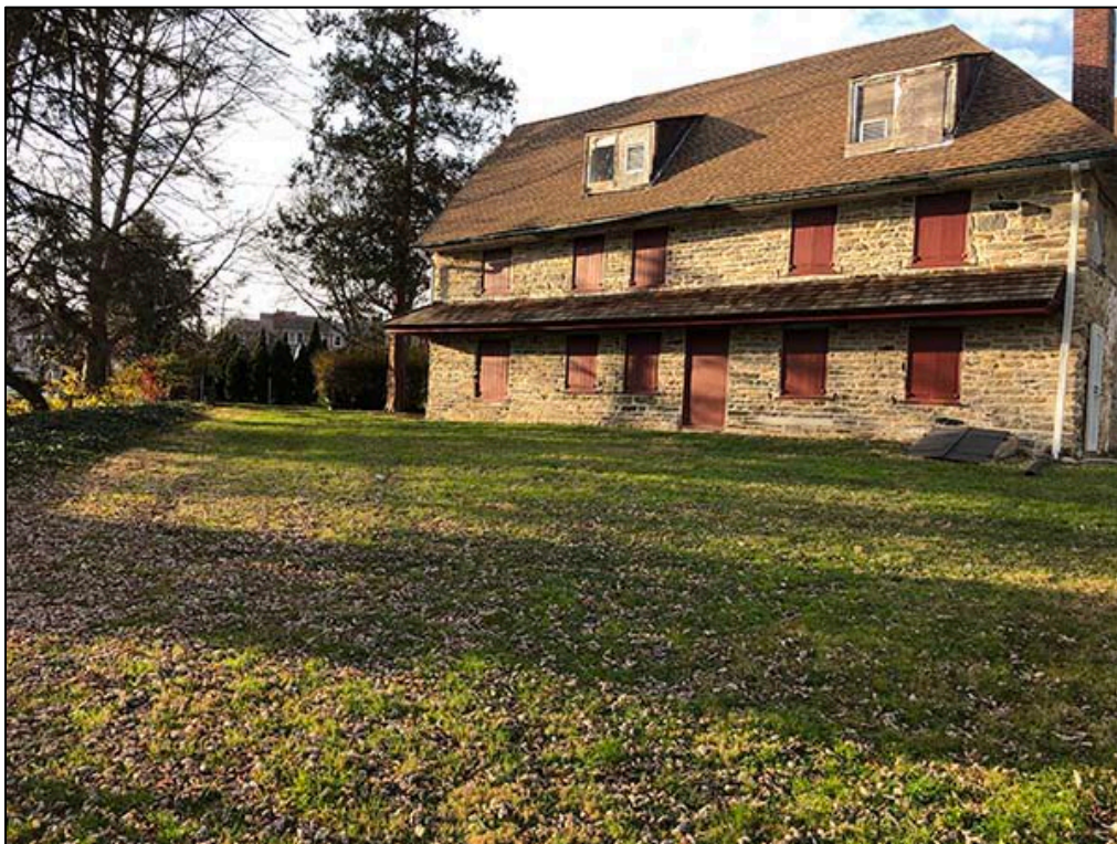
Photograph 1. Overview of the south yard test area from STP A 1, view northwest.
